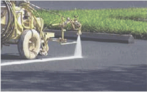
Parking Lot Striping
